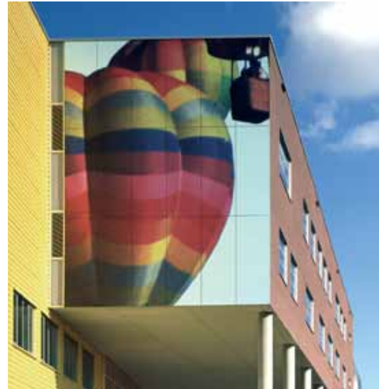
A school in Kerkrade, the Netherlands, by Ector Hoogstad Architects.
