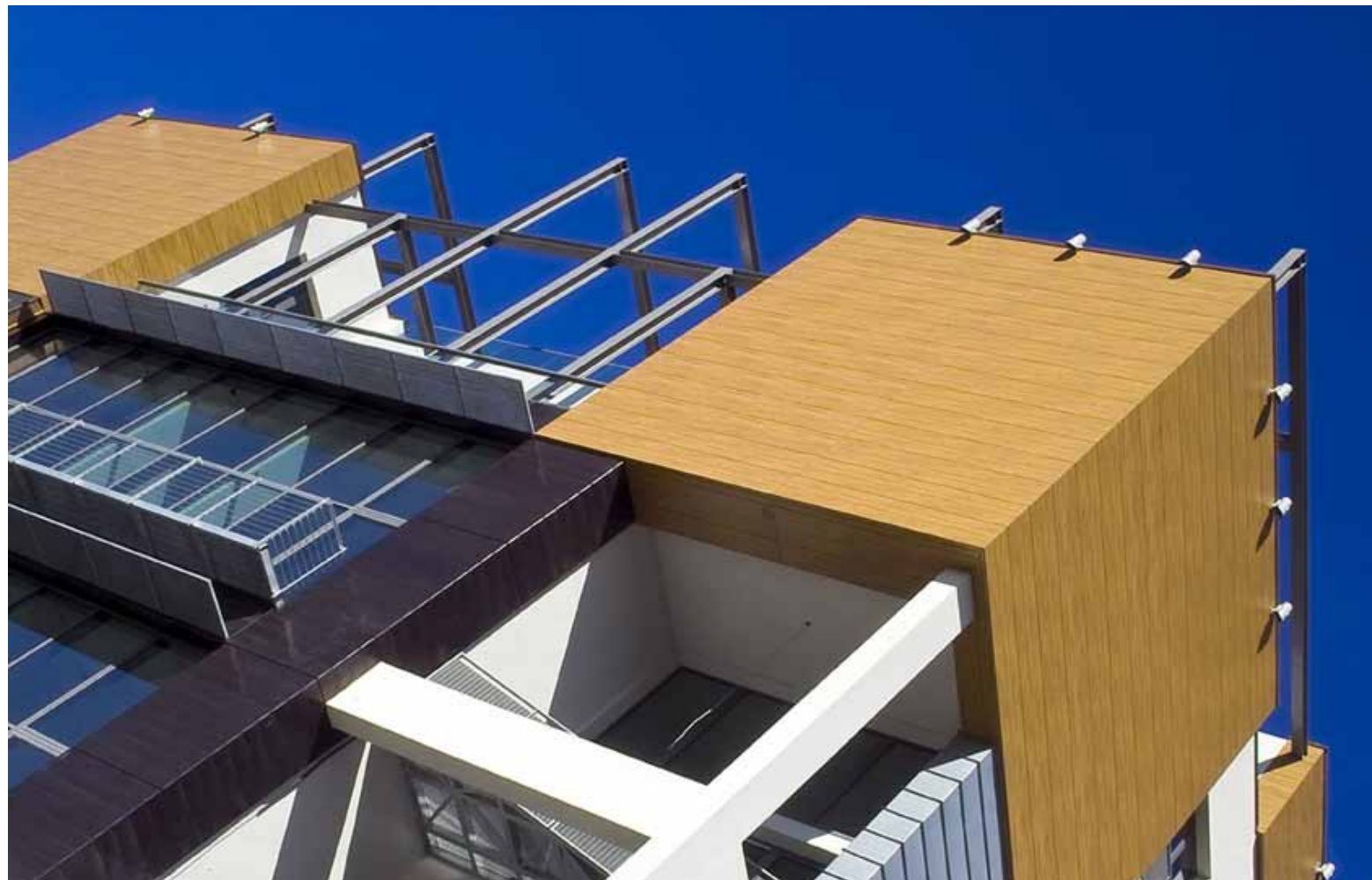
The BIC Building in Brescia, Italy, by Arch. Luciano Grugni.
